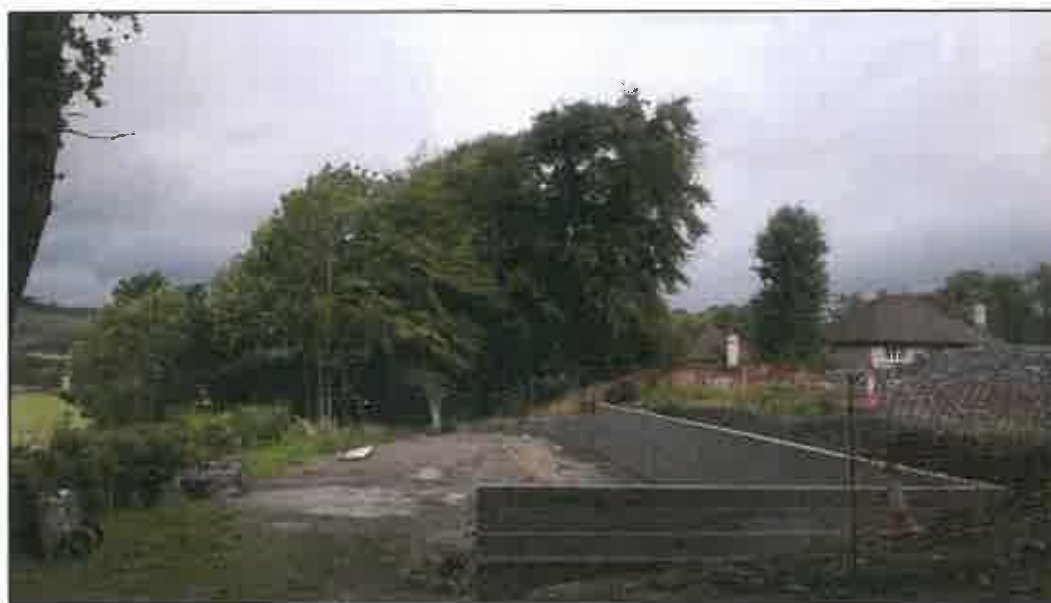
Fig 1: Application Site from the south
